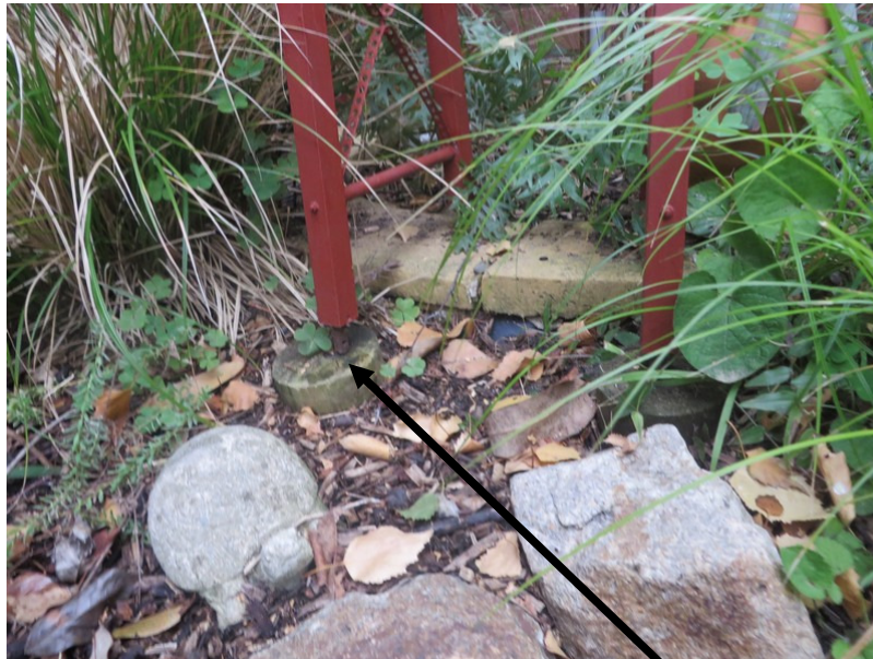
004: Base of steel columns showing adjusting bolt.
